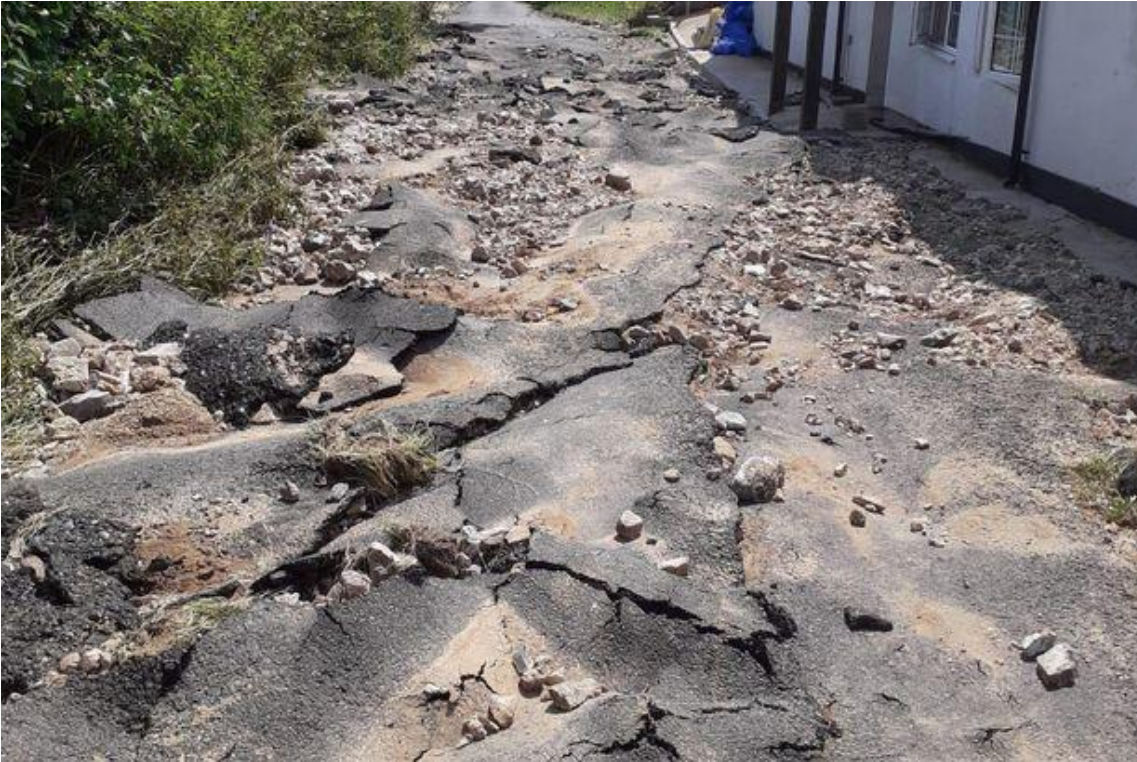
Figure 34: Damage to Scampton lane. From Chard flooding aftermath leaves roads completely destroyed - Somerset Live.
